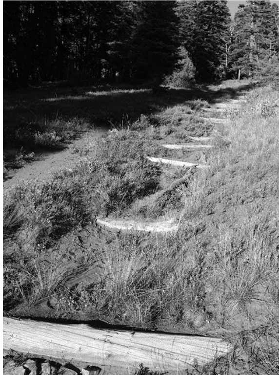
Figure 15: Example of logs used as check dams to help close and restore a section of braided trail.
