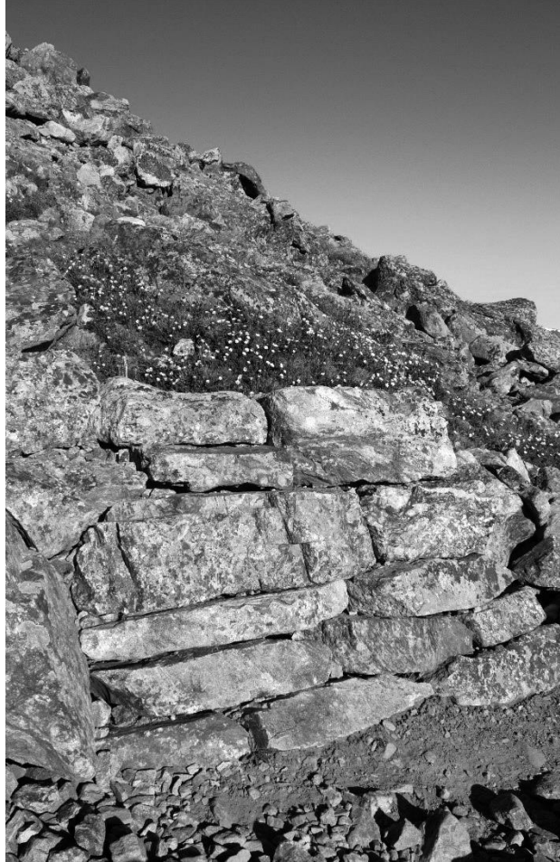
Figure 13: Example of a well-constructed and set back wall supporting Alpine Tundra.
