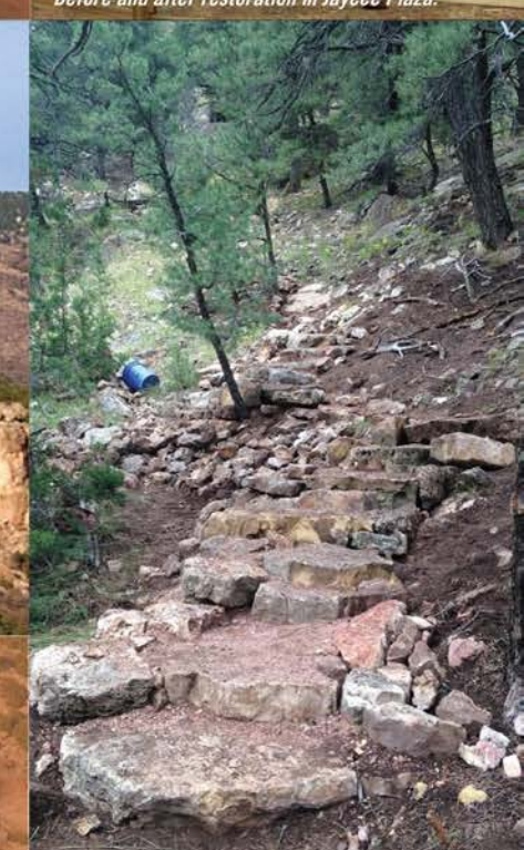
Making sustainable climbing access with rock steps.
