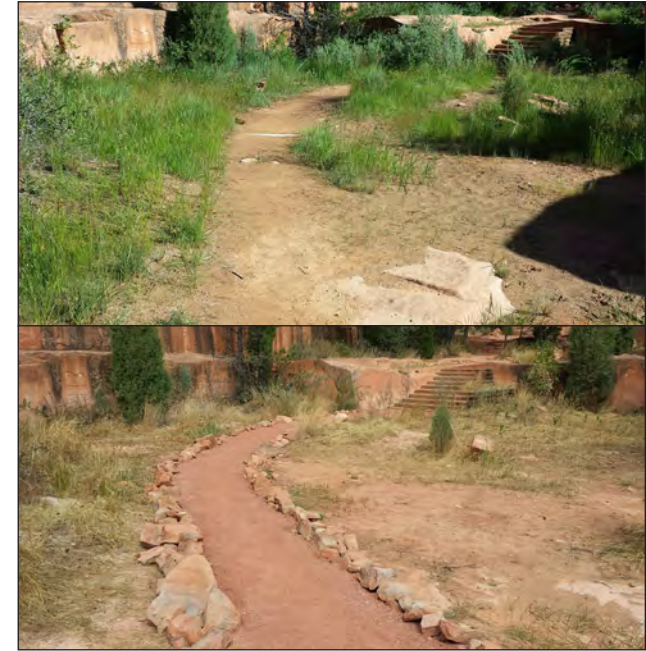
Before and after photos showing repair to a prortion of the Quarry Pass Trail in Red Rock Canyon Open Space.
