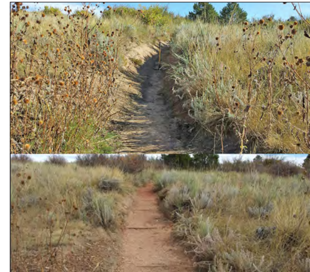
Before and after photos showing results of bringing a deeply incised trail back up to grade in the Garden of the Gods Park.
