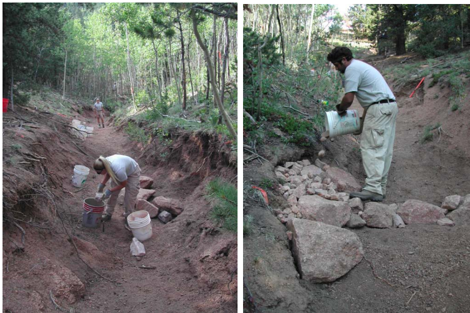
Figure 5 and 6. Examples of building the check dams.
