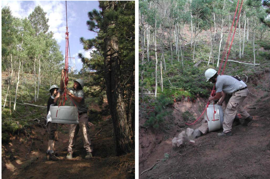
Figure 3 and 4. Examples of unloading the bucket from the tram set up.
