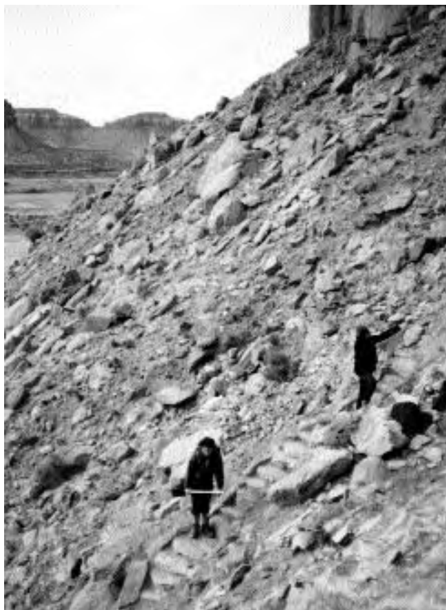
RMFI trail crew completing work on the Cat Wall Trail.
