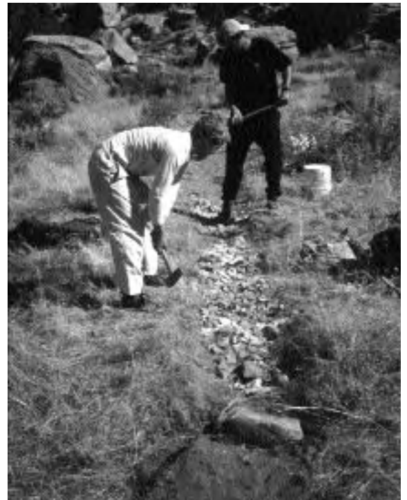
Tread reinforcement
